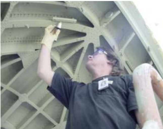
Figure 3 - Operator Applying Conversion Coating Overhead with Touch-N-Prep Pen
